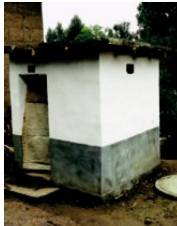
Toilets connected to the tank
